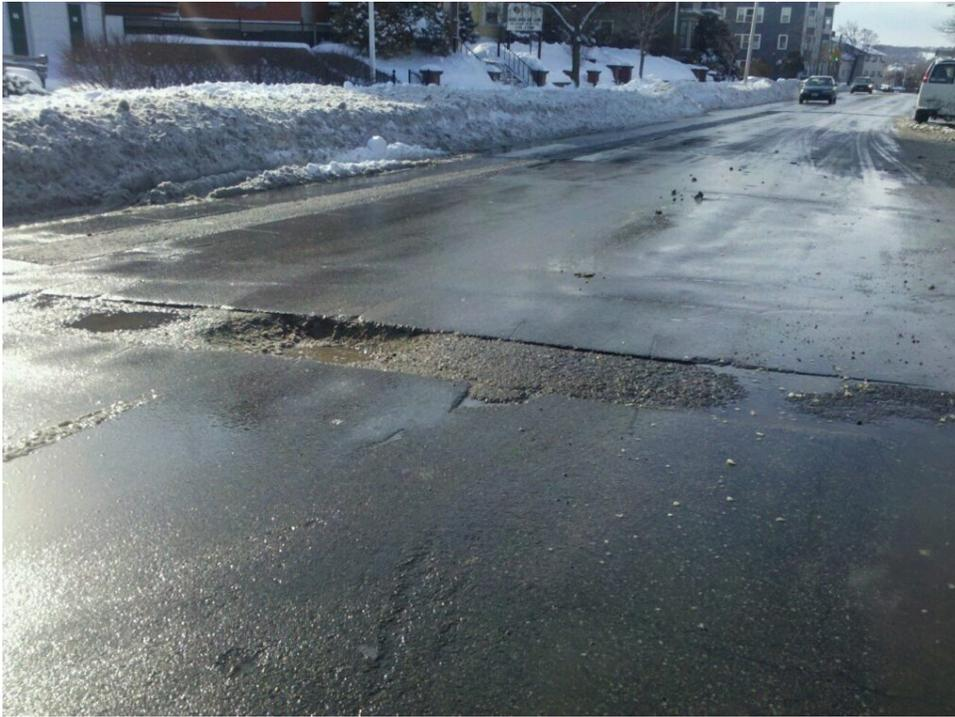
Pothole resulting from utility trench with asphalt patch loosened by snow and rain, looking westward along Westminster St from Bainbridge St in Providence. Jan 27, 2011. (Photo: Michael Bilow)
