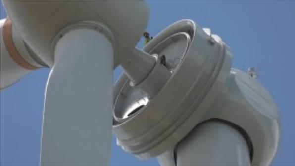
It was not a job for anybody with a fear of heights. More than 400 feet up, workers headed into the homestretch assembling a 1.5 megawatt wind turbine in western Coventry. A crane operator on the ground and a supervisor at the top worked together to maneuver the blades into place. Each blade weighs nine tons and measures 134 feet. The fit has to be exact.
